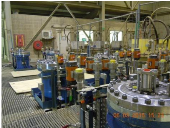
Budel: Newly installed and operational TPF filters
