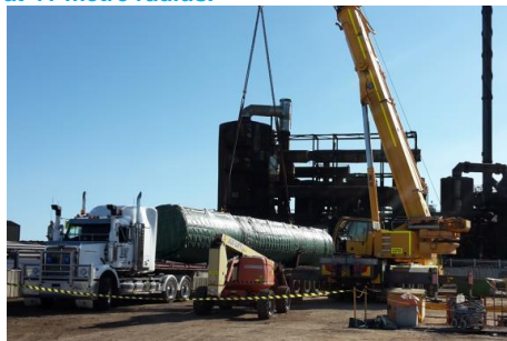
Unloading section II of the Stack. One of four sections of the 60-meter high Stack.
