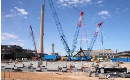
Work continues on the HPDE liner which stops acid entering the ground and underlying aquifers from leaks or spills.
