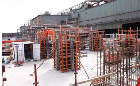
Setting up of the TSL Furnace footings
