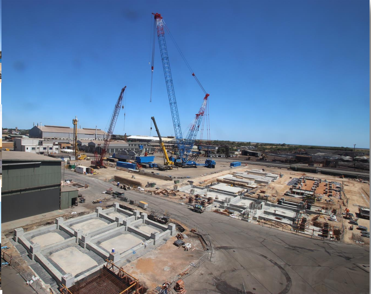
Assembly of the 2600 tonne heavy lift crane commences. Lift capacity of 1084 tonnes at 41 metre radius.
