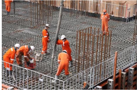
720 cubic metre concrete pour at the southern end of the TSL foundation.
