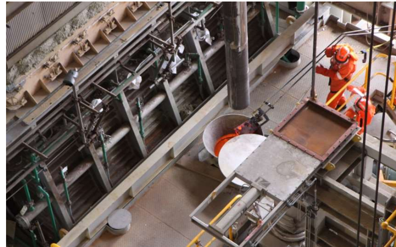
New slag launders installed – October 2017
